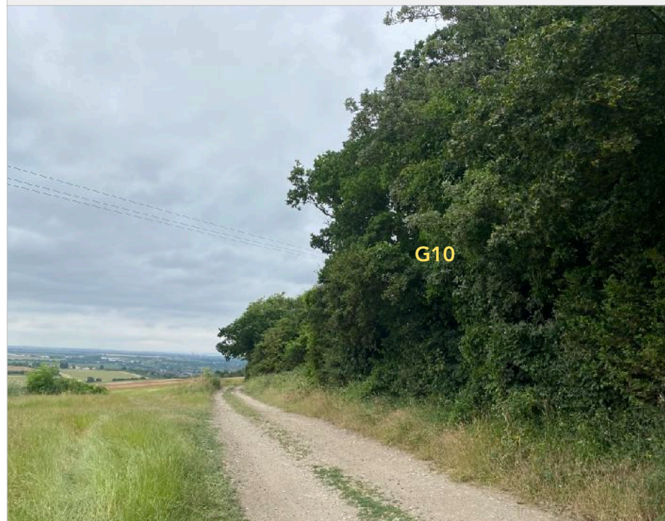
IMAGE 4: Existing compacted earth and stone track through the centre of the site.
